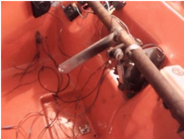
TUBE HELD IN PLACE; ARM WELDED IN PLACE
